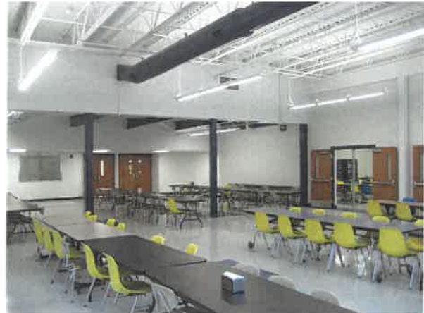
Clay County High School Renovation LED Replacement Lighting
