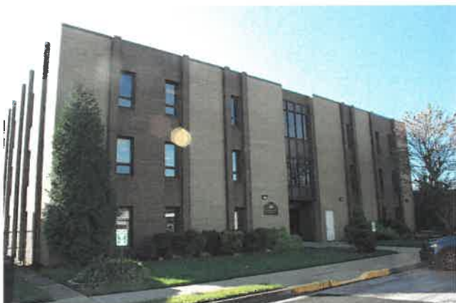
Building 74 was to be renovated while occupied.
