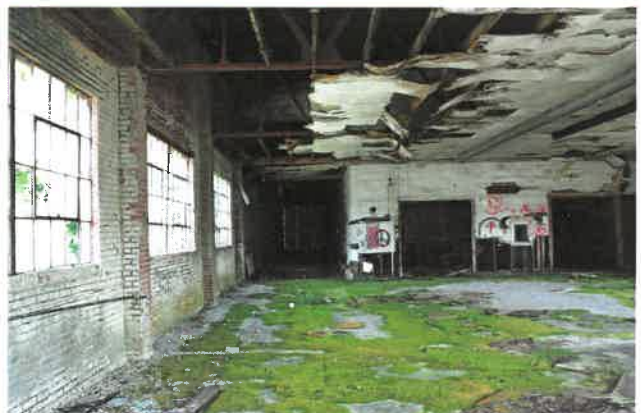
Right: Interior prior to renovation.
