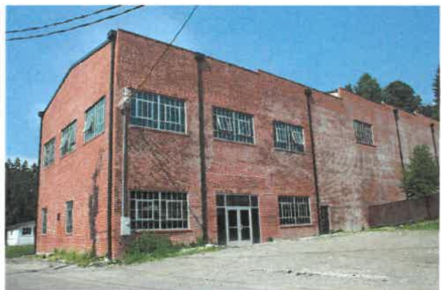
Coal Heritage Center after window replacement.
