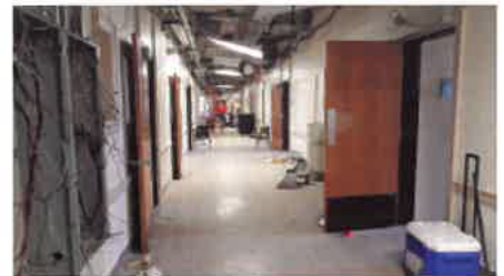
Above: Early Demolition
