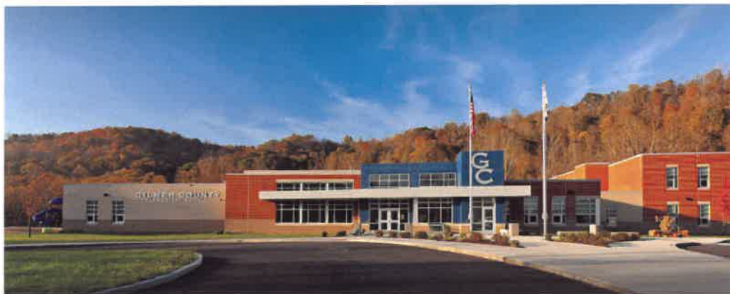
At left LEED Silver Certified Gilmer County Elementary School in Glenville, WV featuring energy efficient Insulated Concrete Form (ICF) wall systems, white EPDM roofing and located on a Brownfield Reclamation site. Gilmer County Elementary School is Williamson Shriver Architects' third LEED school project.
