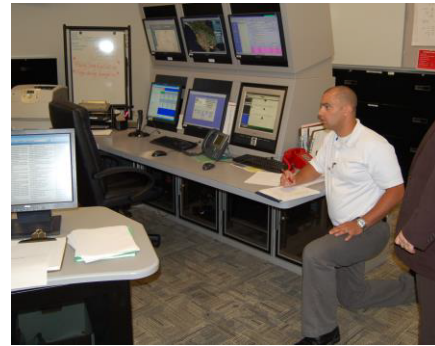
Matthew Allain, Project Resource, conducts an assessment of a security control room for equipment upgrades.
