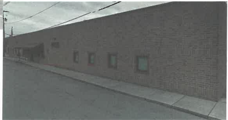
Building 97 - DHHR Slab Repair
