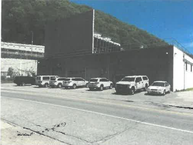
Building 11 - Chiller Plant Wall Repair
