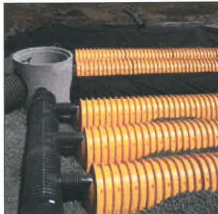
Underground Stormwater Storage
