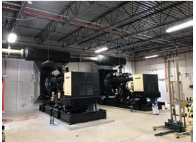
incorporates planned upgrades from the local utility authority which will be a transition from 4160 V to the 13.2 kV. Functional areas with the PPB include space allocation of the 2 generators with reserved interior floor space for future generator growth, and integration with alternate energy systems within the National Guard Training Center installation (Photovoltaic, wind, storage) using parallel switchgear and control interfaces.
