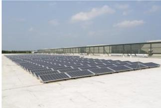
*NJARNG AASF Hangar Roof Mntd. PV Panels generate 207kW of power*
