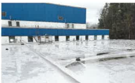
Progress photos of the 2019 roof replacement at Lewis County High School
