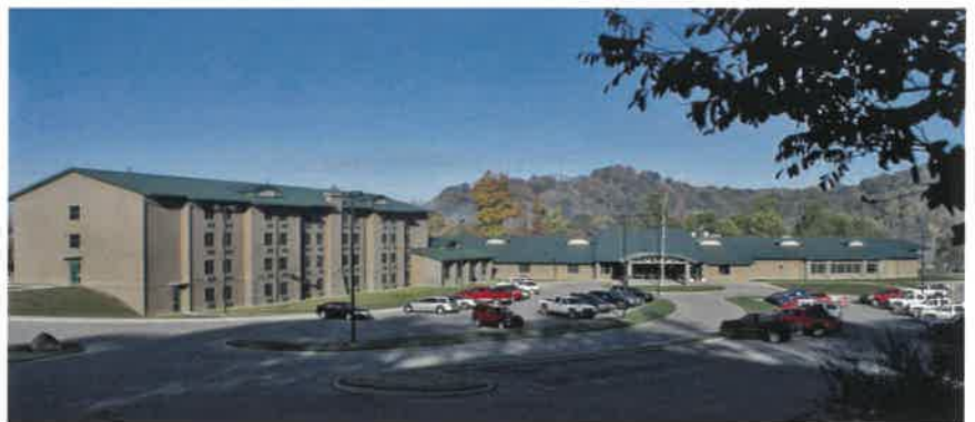
Above: Front facade of the Chief Logan State Park Lodge. The right conference center was completed in 2002 and the left guest suite addition was complete in 2006
