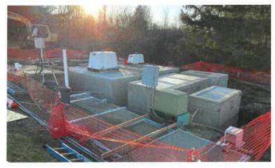
WWTP to increase ease of operation during the winter months. A new grease trap, new gravity sewer lines, and new manholes were constructed and tied-in to the existing sewer lines.
