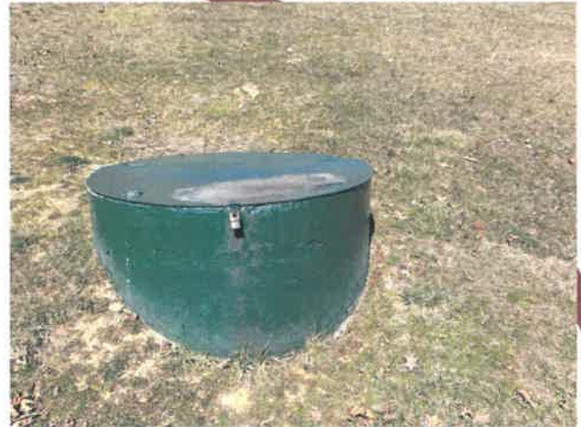
Village Sanitary Board Wastewater System's Sewer cap (end of the line) above; and roadside sewer cleanouts below. All photos by Dunn Engineers, Inc.
