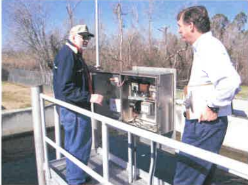
Mr. Hypes (left) as consulting engineer at a wastewater treatment plant in Mississippi after Hurricane Katrina.
