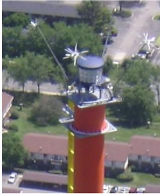
are either horizontally or elliptically polarized include a galvanized steel climbing pole for beacon access. All top mounted TRASAR antennas include four (4) lightning spurs at the top of the antenna.
