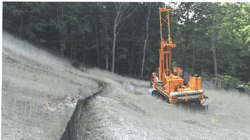
Drilling on Landslide
