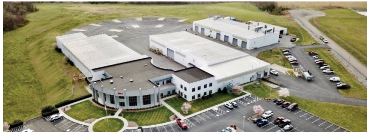
Figure 1-4. Bell Piney Flats Service Center.
