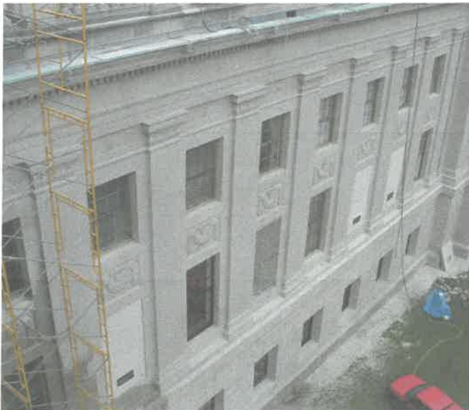
Exterior façade restoration included cleaning, pointing, and repairs to the limestone and terra cotta components, windows and doors.
