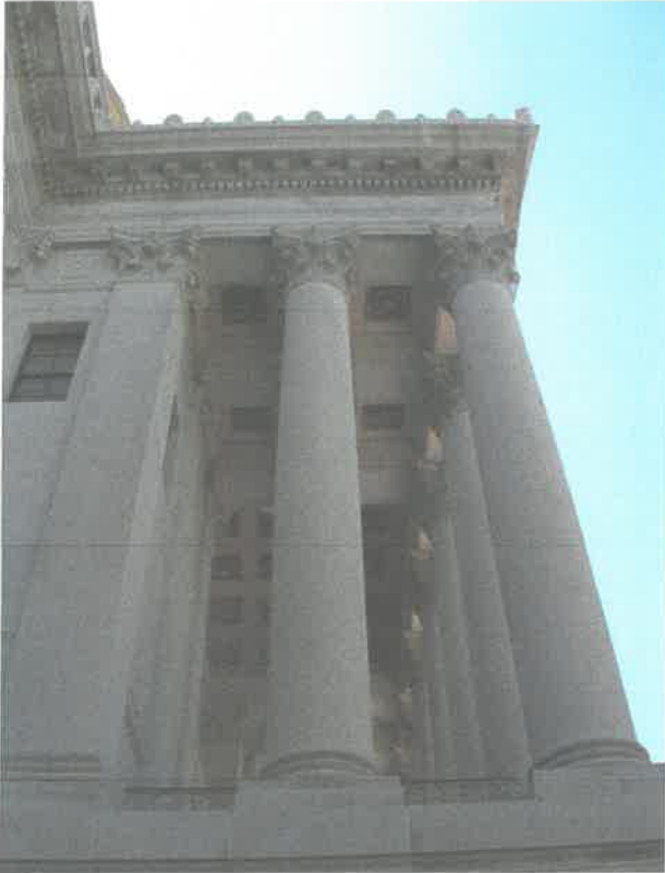
Exterior façade restoration included cleaning, pointing, and repairs to the limestone and terra cotta components, windows and doors.
