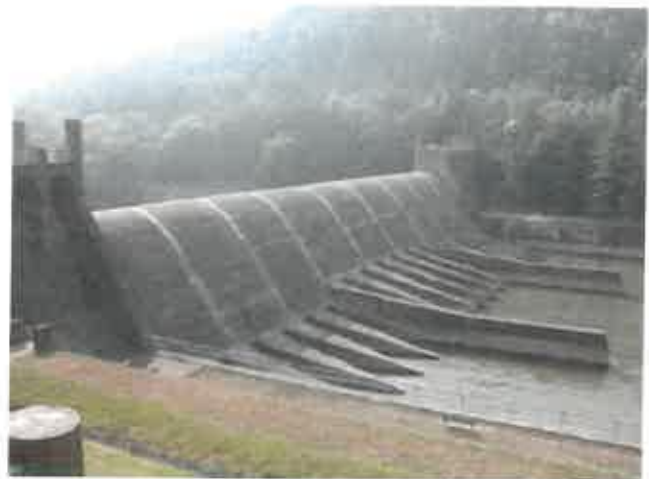
Dover Dam, OH. Foundation Stabilization 2014
