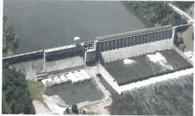
Bluestone Dam, Hinton, WV. Foundation Stabilization
