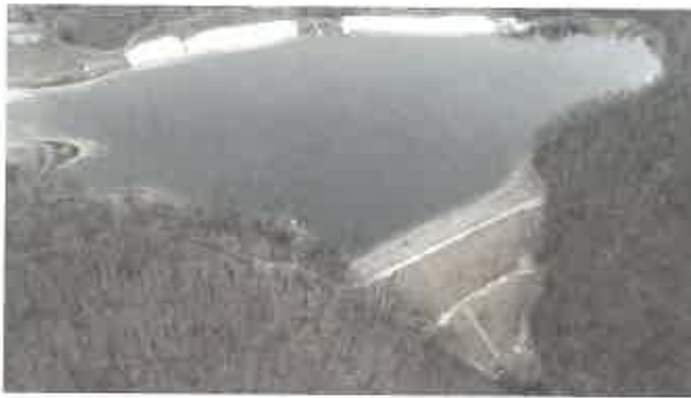
An unmanned aircraft survey (UAS) was performed of the dam, dike, spillway, reservoir and access roads.
