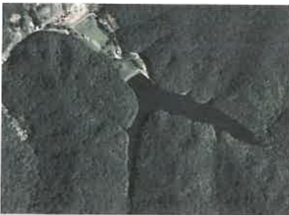
Beech Creek Dam and the impounded lake are the primary water supply facility for the City of Manchester, Kentucky.
