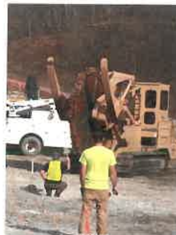
Trenching in the bedrock for the foundations of the walls.
