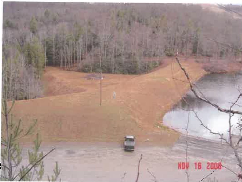
PLUM ORCHARD DAM MODIFICATION, FAYETTE CO., WV
