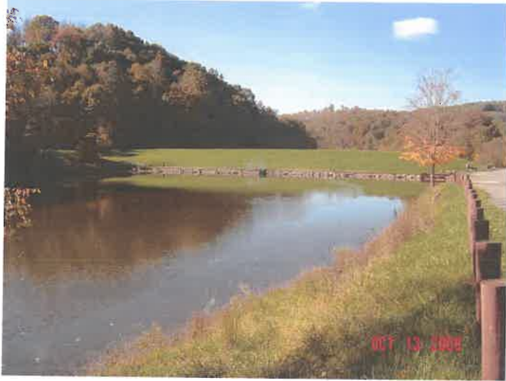
JIMMY LEWIS DAM MODIFICATION, MERCER CO., WV
