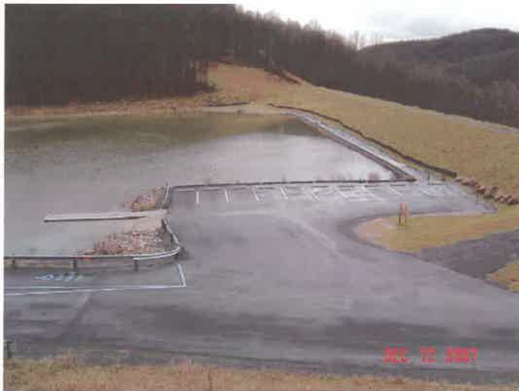
BAILEY DAM MODIFICATION, MONONGALIA CO., WV
