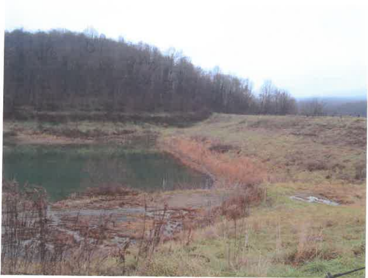
BAILEY DAM MODIFICATION, MONONGALIA CO., WV (BEFORE)
