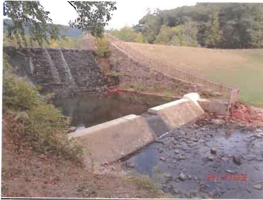
PARK DAM MODIFICATION COMPLETE, CACAPON STATE PARK
