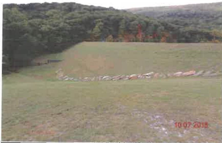
RESERVOIR DAM MODIFICATION, CACAPON STATE PARK (BEFORE)
