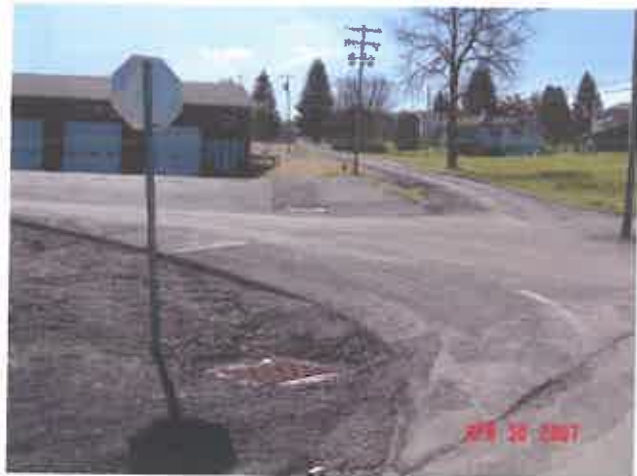
New Storm Drains and Catch Basins
