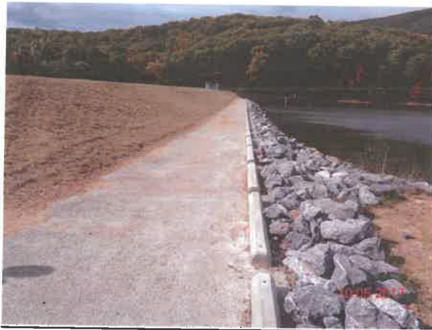
RESERVOIR DAM MODIFICATION, CACAPON STATE PARK (AFTER)
