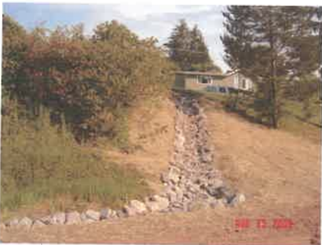
Erosion Repair – Rip Rap Armored Ditch
