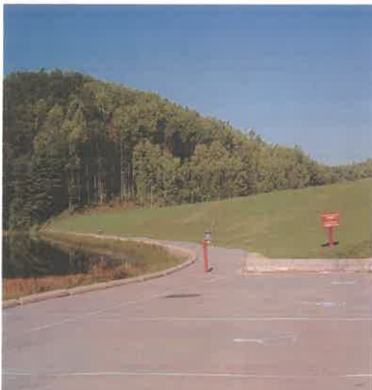
TETER CREEK DAM MODIFICATION, BARBOUR CO., WV
