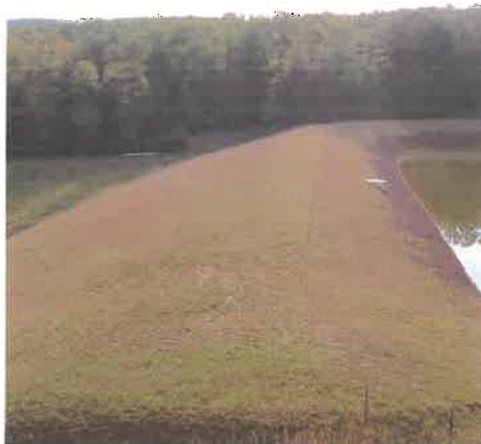
WILSON DAM MODIFICATION, HAMPSHIRE CO., WV
