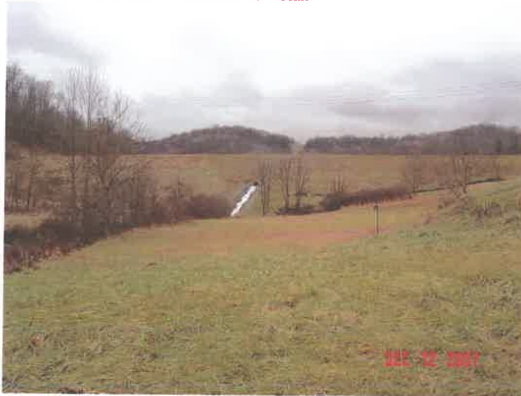
LEMLEY DAM MODIFICATION, MONONGALIA CO., WV
