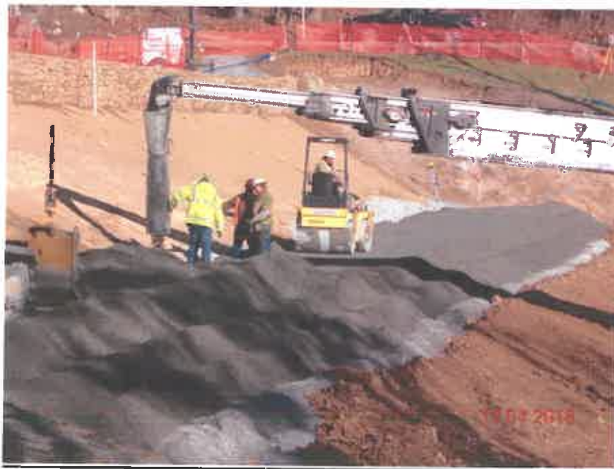
PARK DAM MODIFICATION (RCC PLACEMENT), CACAPON STATE PARK
