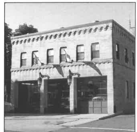
Central Fire Station
