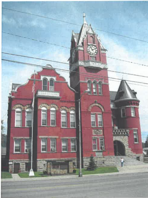
Tucker County Commission Jailer's Residence Restoration 213 First Street Parsons, West Virginia
