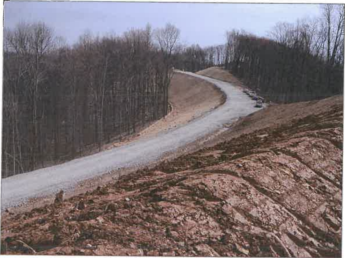
New Access Road to Well Site in Doddridge County, WV
