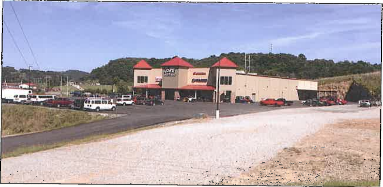
Site and Building Near Completion
