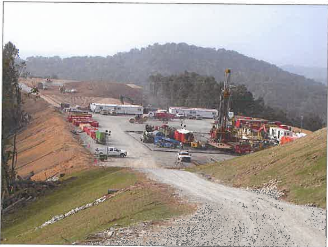
Access Road and Operating Drill Pad in Wetzel County
