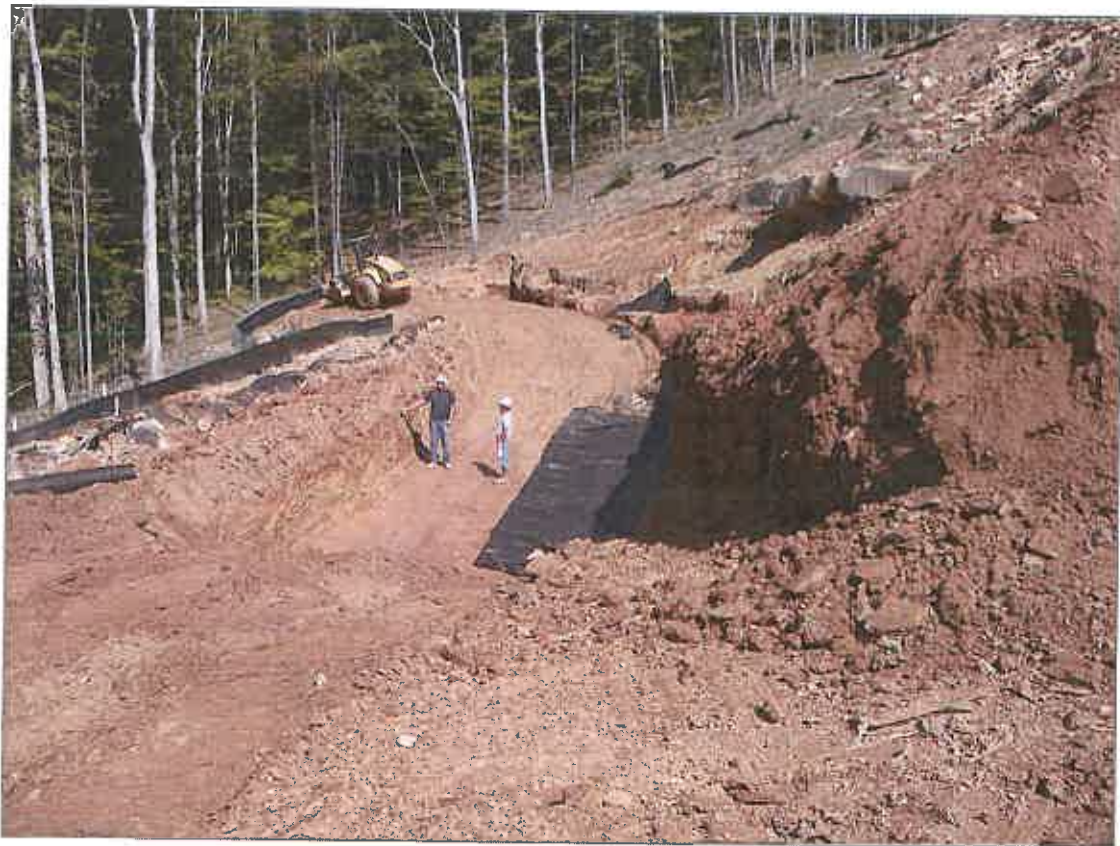
Embankment Fill Keyway for Impoundment Site in Doddridge County, WV
