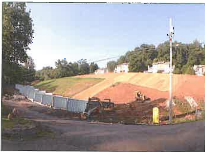
Initial Site Development
