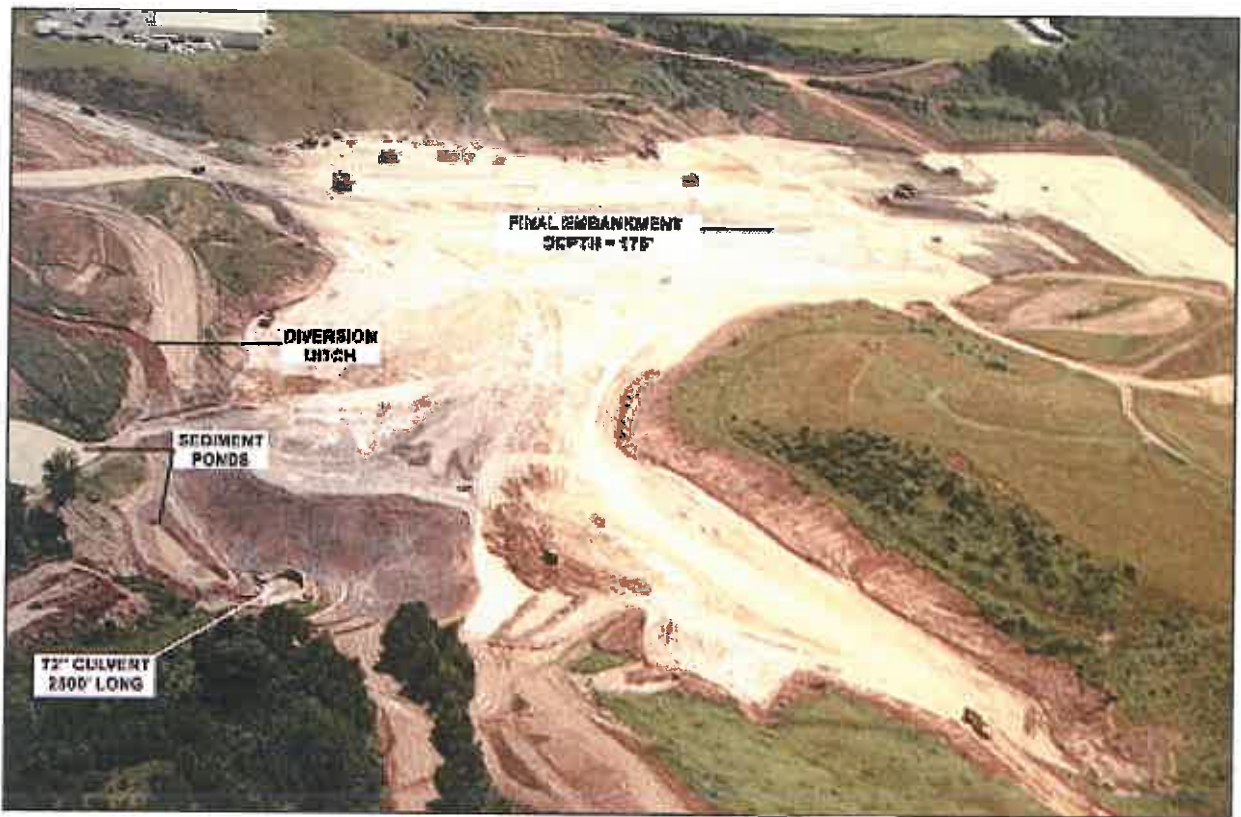
BENEDUM AIRPORT RUNWAY EXTENSION PROJECT
