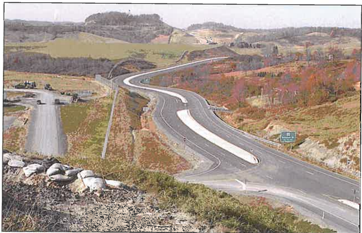
ROUTE 279, NORTH BRIDGEPORT BYPASS
