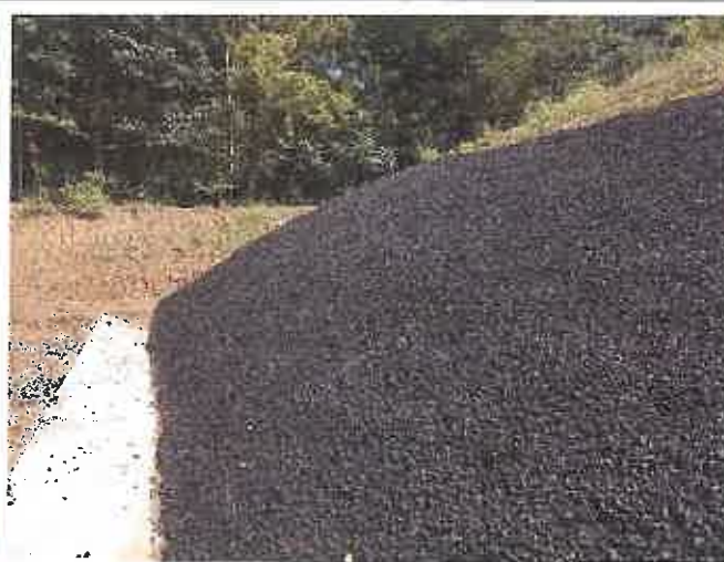
Granular Rubber Bullet Trap after renovation
