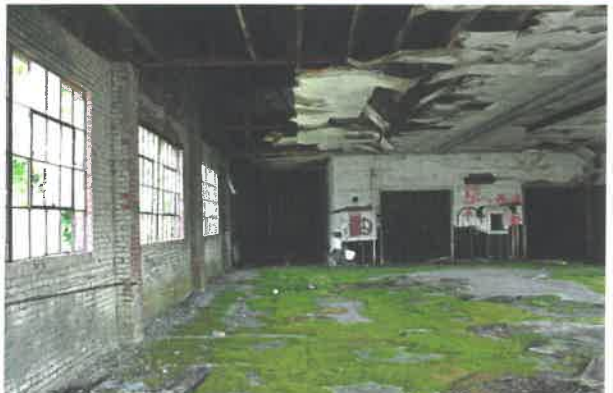
Right: Interior prior to renovation.
