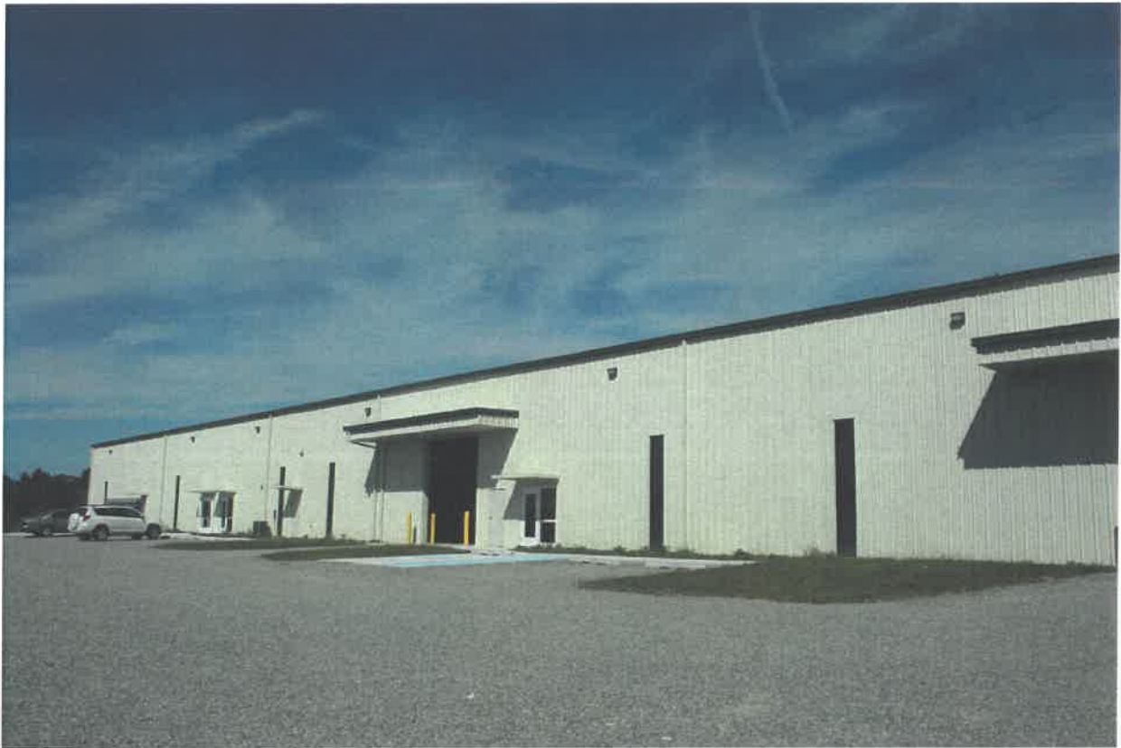
Barbour County Economic Development Authority Belington Multi-Tenant Business Incubator Belington Industrial Park Belington, West Virginia
