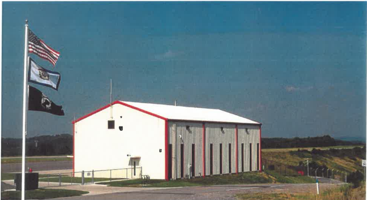
Buckhannon-Upshur County Airport Snow Removal Equipment Building 38 West Main Street Buckhannon, West Virginia
