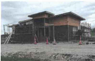
New Terminal Building Jackson Airport
