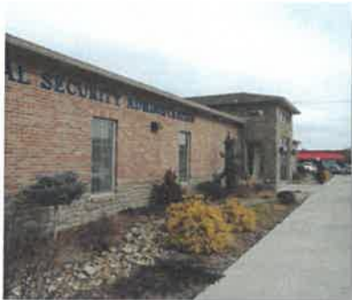
Portsmouth Social Security Administration Office
