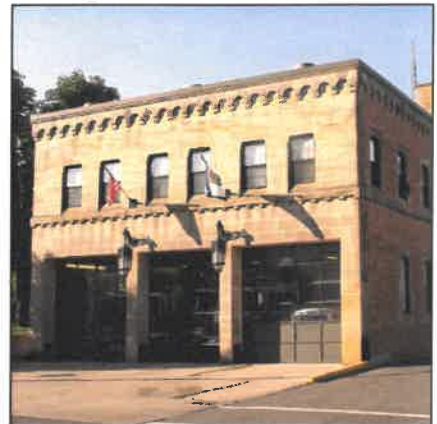
Central Fire Station
