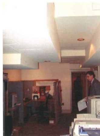
Fig 6: Multiple Bulkheads and Access Panels at 4 th Floor
