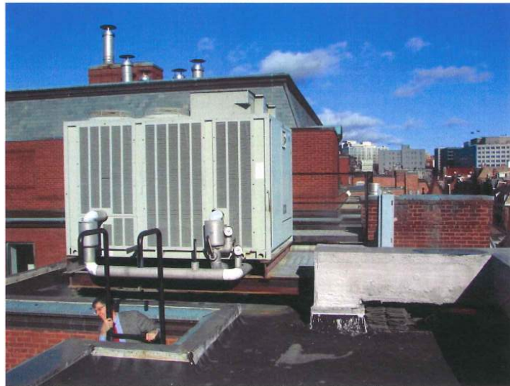
Fig 1: Air Cooled Chiller on Roof of House Building (nominal 60 tons)
