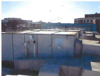
Fig 4: Air Handling Units on Roof
