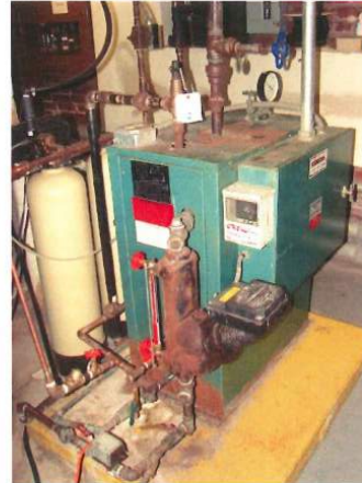
Fig 3: Electric Humidification Steam Boiler
