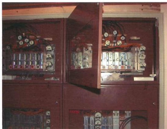
Fig 11: Antiquated Honeywell Pneumatic Control Panel
