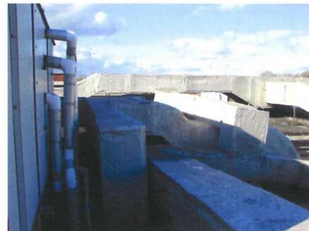
Fig 5: Ductwork on Roof Impedes AHU Access
