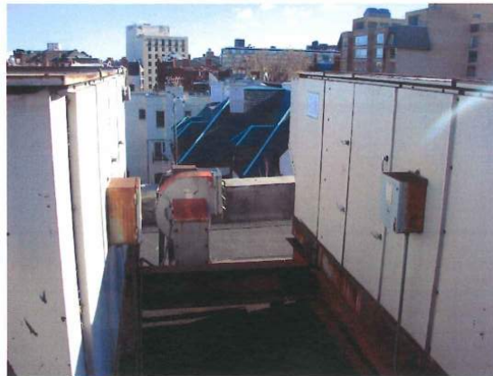
Fig 10: Toilet Exhaust Fan Discharging at AHU Inlet
