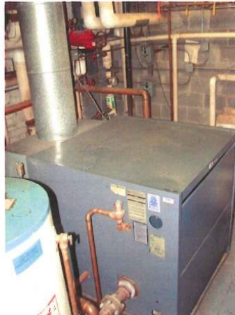
Fig 2: Cast Iron Heating Water Boiler
