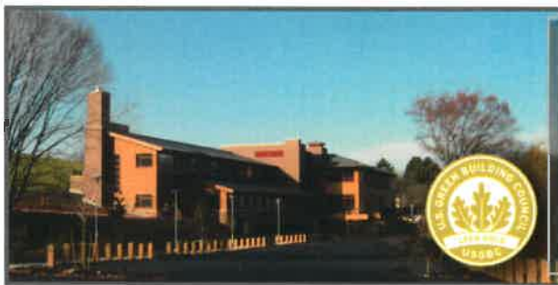
Harvard University Arnold Arboretum Weld Hill Research and Administration Building
