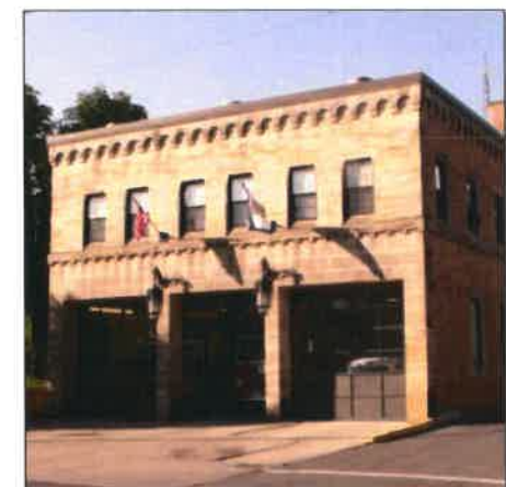
Central Fire Station
