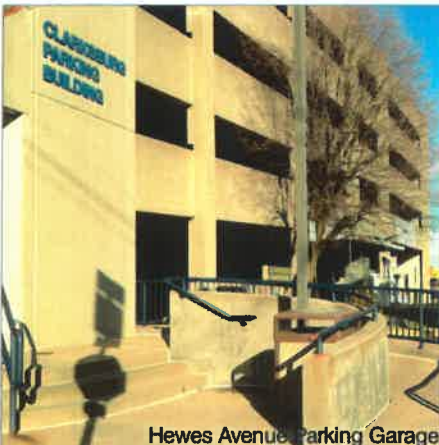
Hewes Avenue Parking Garage
