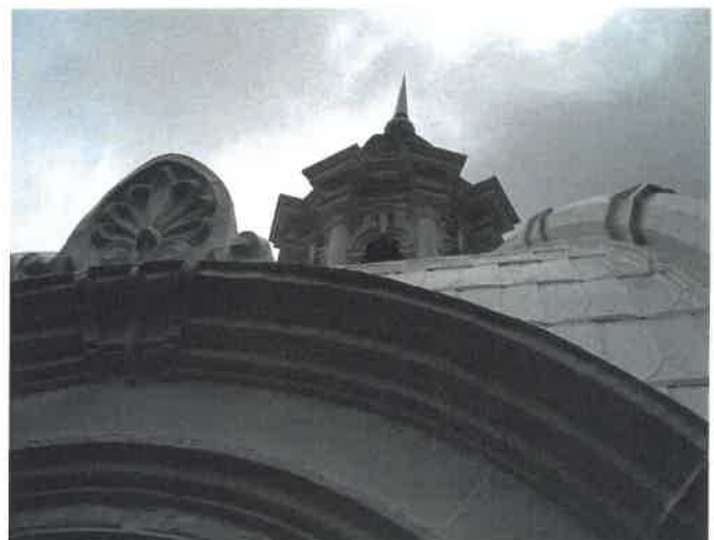
Dome Restoration Detail
