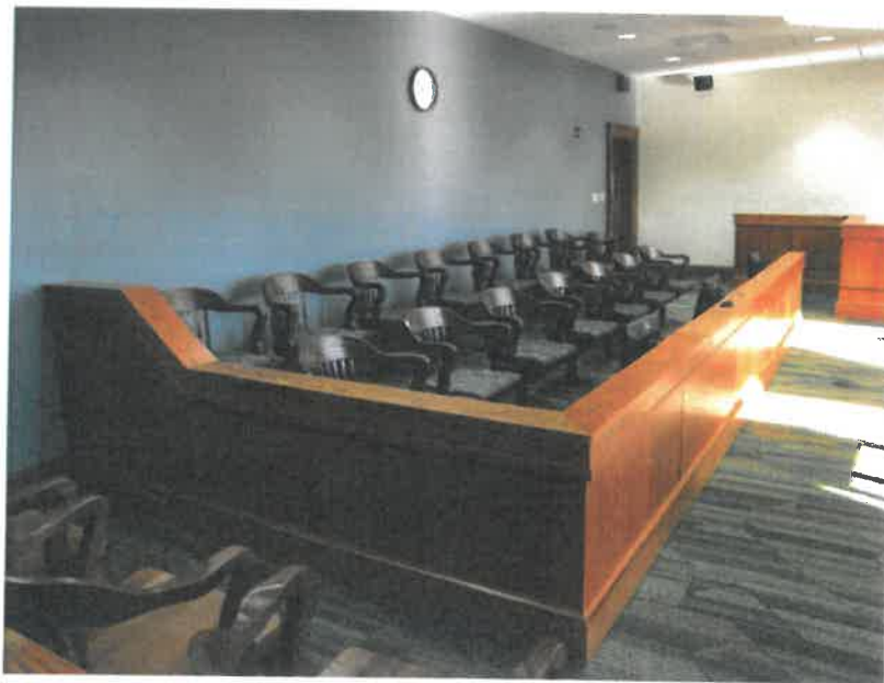
The expanded jury box included a new low wall to match existing millwork, and new pedestal base chairs in the period style.
