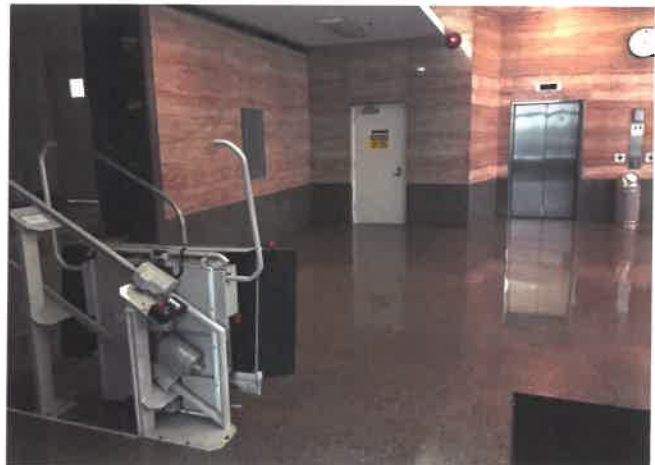
Existing West Stair Life for Building Four presents an awkward, architecturally incompatible means to move from the Lobby to First Floor.
