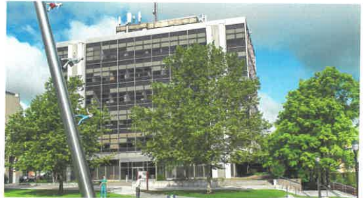
Warner Hall Admin. Building Renovation, Carnegie Mellon, Pittsburgh, PA
