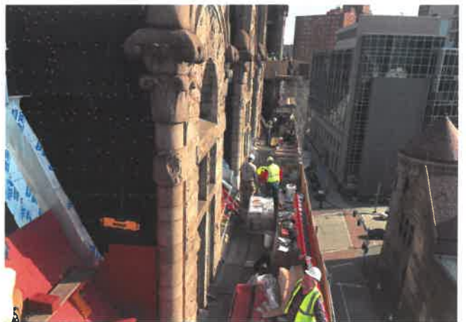
The scaffold platform doubles as a staging area for materials.
