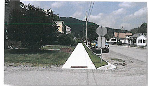
Parsons Sidewalk Improvements
