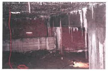
The deteriorated concrete was removed, galvanized metal deck was put in place and a new reinforced concrete slab was poured.
