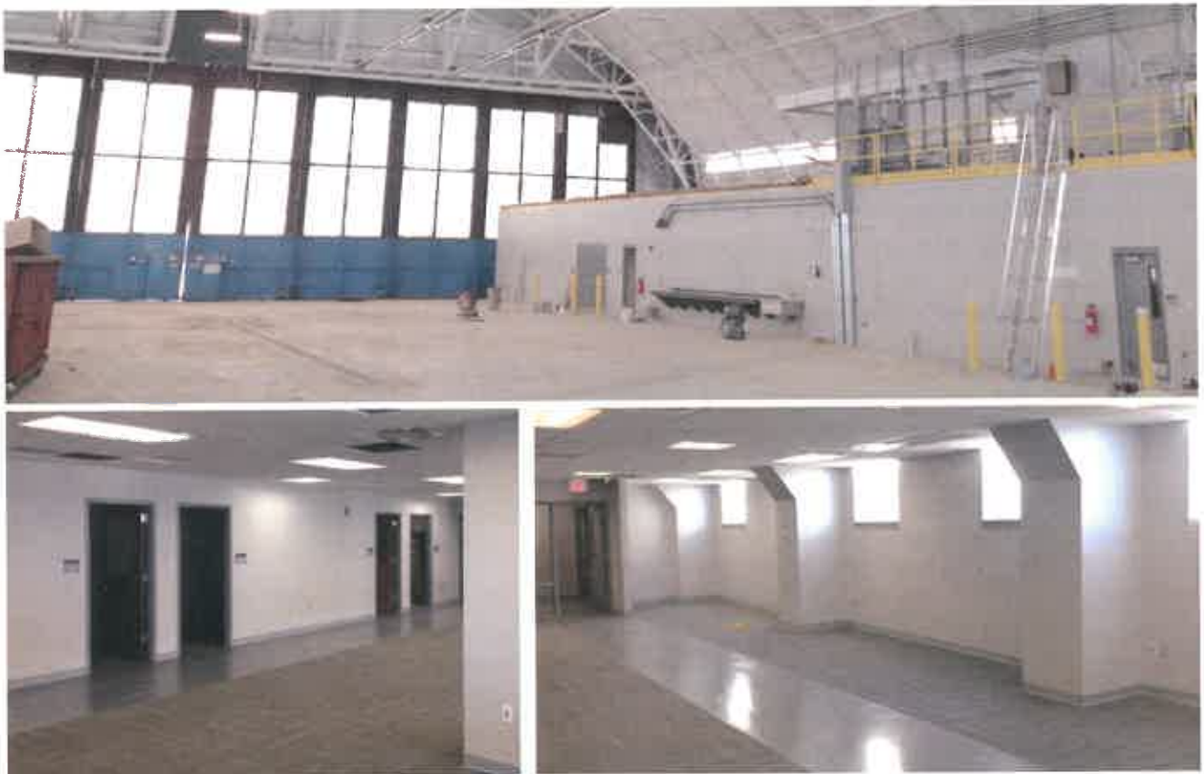
GRW provided design and construction phase services for the WV ANG's 130 th Airlift Wing Building 107 Renovation. With a construction budget of $5M, the awarded bid was $4,941,290, and the final construction cost was $4,991,876 (within 1% of awarded bid).
