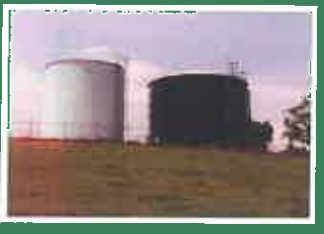
Alderson Water Storage Tanks
