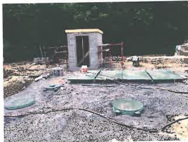
Installation of Orenco treatment units
