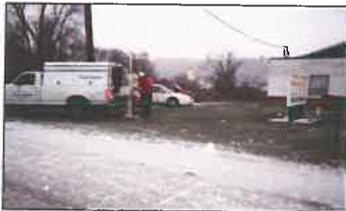
Soil Boring During Limited Phase II ESA
