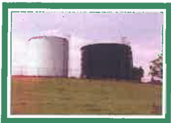
Alderson Water Storage Tanks
