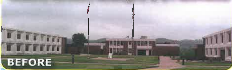
Academy Dormitory Buildings A, B, & C Renovations
