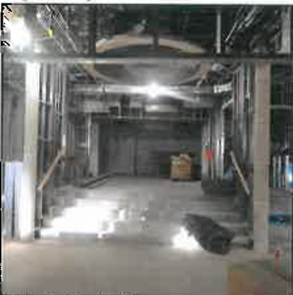
Lobby - In Construction
