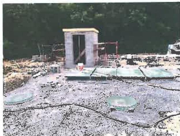
Installation of Orenco treatment units
