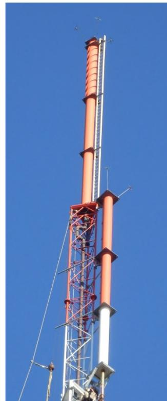
ERI TRASAR UHF Television Antennas. Both the antennas pictured are elliptically polarized UHF antennas. One is top mounted on a lattice pedestal designed and built by ERI and a side mounted UHF TRASAR Antenna is mounted on one face of the pedestal.
