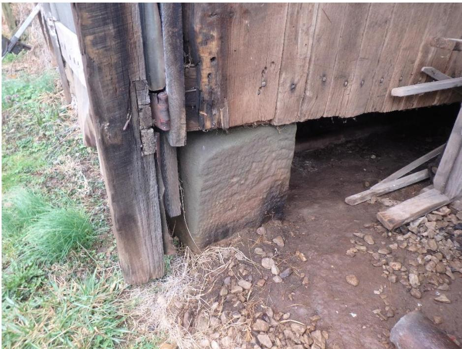
Photo 14. Original exterior wall of barn, note cut stone pier and square nails (looking north).
