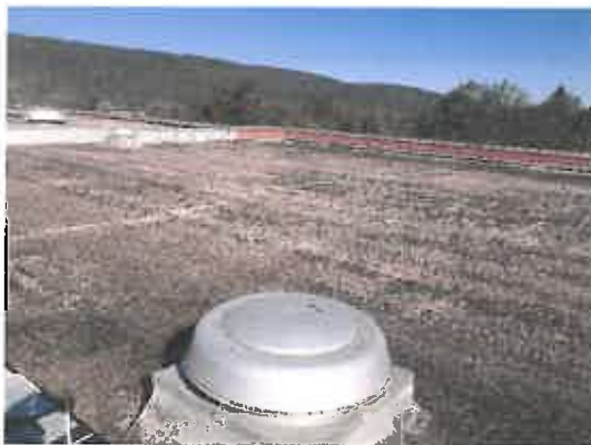
School for the Deaf - Roof
