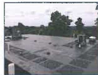
WVU-Tech Classroom Roof
