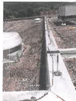
Roof Top Curb
