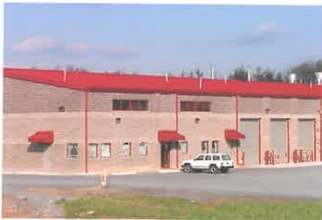
DISTRICT 10 MAINTENANCE BUILDING
