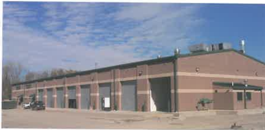
DISTRICT 6 MAINTENANCE BUILDING
