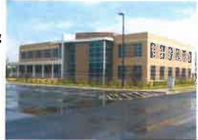
Beltzel Office Building Grantsville, MD
