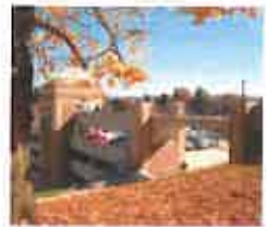
Fairmont State University Parking Garage Fairmont, WV
