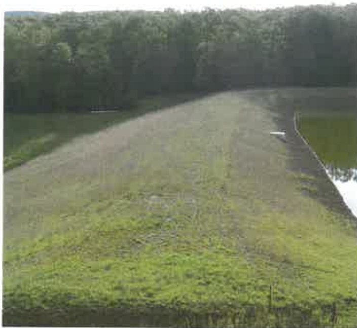
WILSON DAM MODIFICATION, HAMPSHIRE CO., WV
