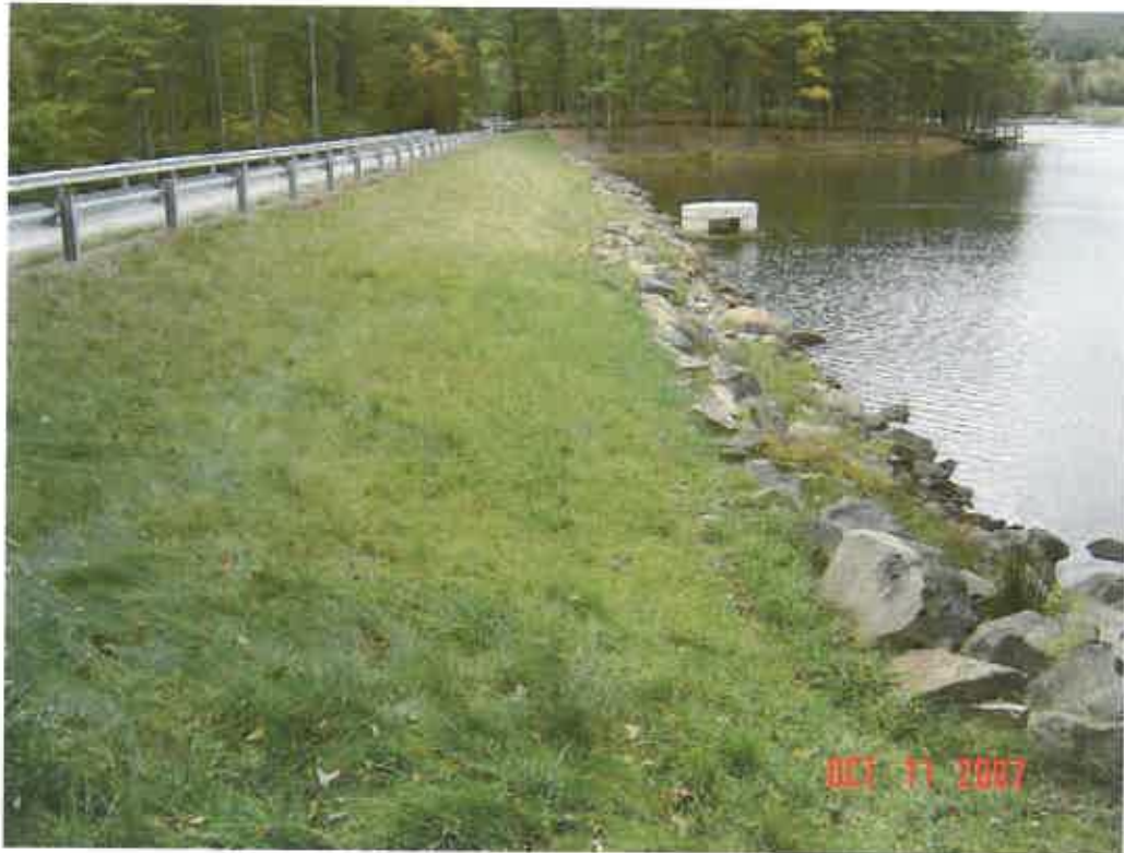
MONCOVE DAM MODIFICATION, MONROE CO., WV
