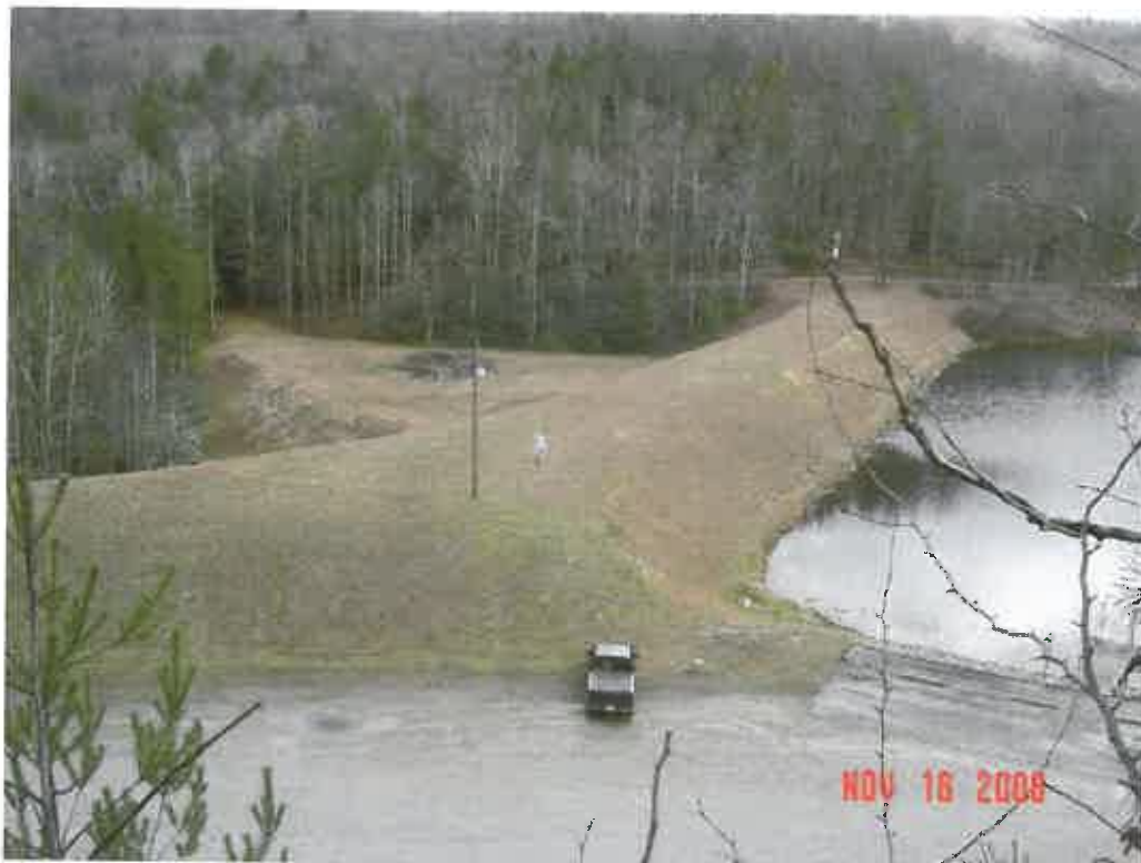
PLUM ORCHARD DAM MODIFICATION, FAYETTE CO., WV
