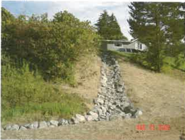
Erosion Repair – Rip Rap Armored Ditch
