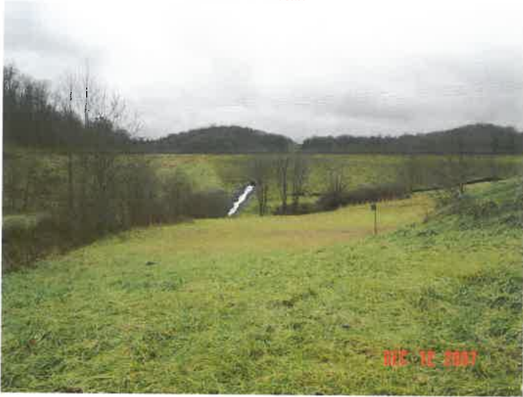
LEMLEY DAM MODIFICATION, MONONGALIA CO., WV
