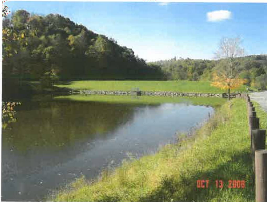
JIMMY LEWIS DAM MODIFICATION, MERCER CO., WV
