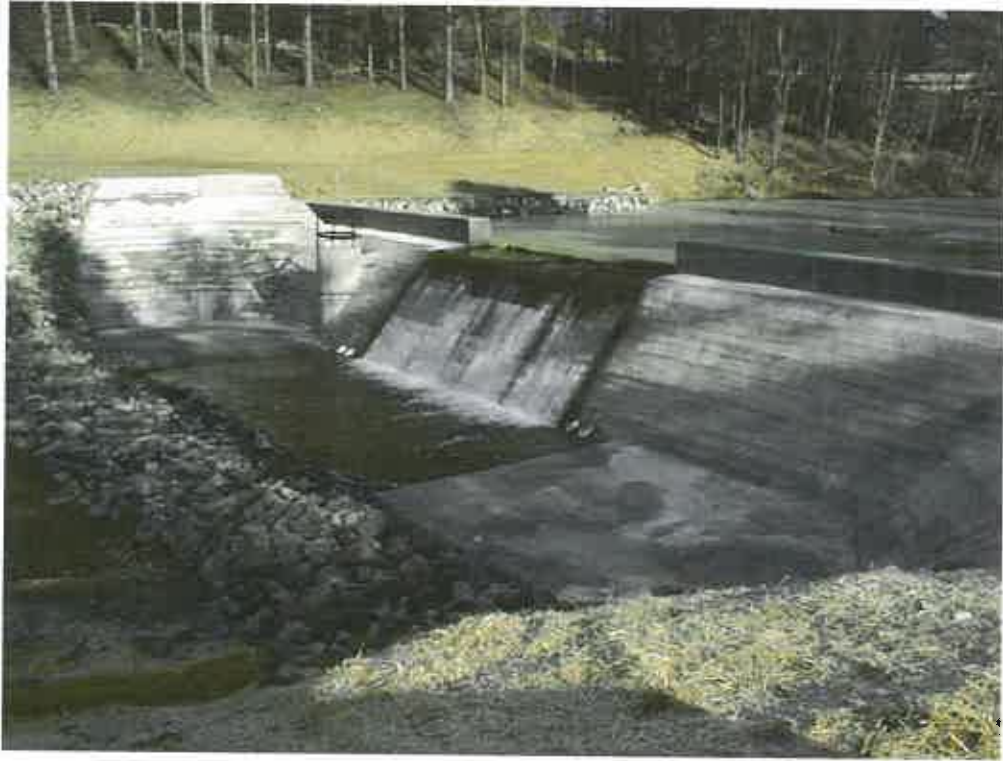
THOMAS DAM MODIFICATION, THOMAS, WV
