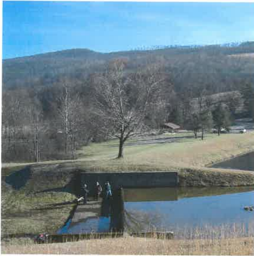
BELINGTON DAM MODIFICATION, BELINGTON, WV
