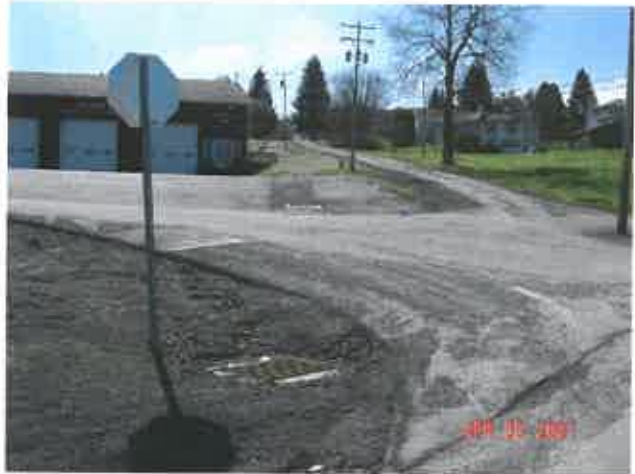
New Storm Drains and Catch Basins
