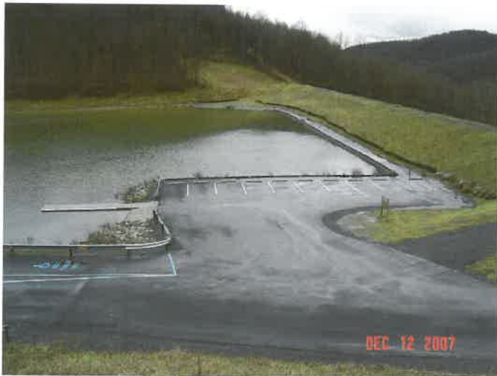
BAILEY DAM MODIFICATION, MONONGALIA CO., WV
