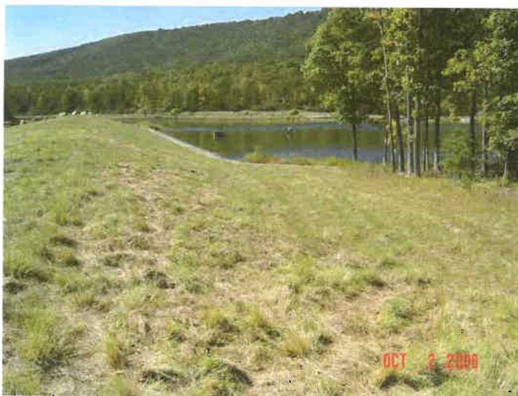
WARDEN LAKE DAM MODIFICATION, HARDY CO., WV
