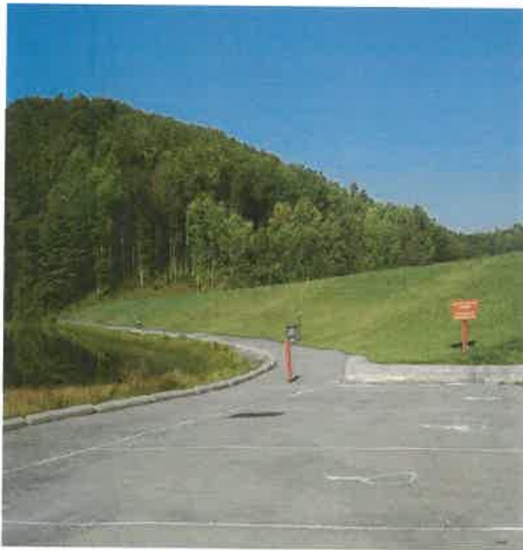
TETER CREEK DAM MODIFICATION, BARBOUR CO., WV
