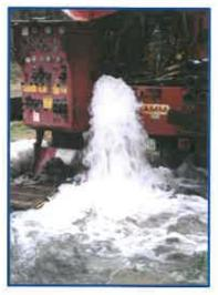
The "bubbler" borehole has an estimated flow of 500 gallons per minute (gpm). It had been cased and connected to a piping system for transport of the collected acid mine drainage to an existing passive treatment system. The borehole casing had been leaking for several years, and due to the artesian flow conditions, required replacement and abandonment to prevent direct discharges to the adjacent stream.
