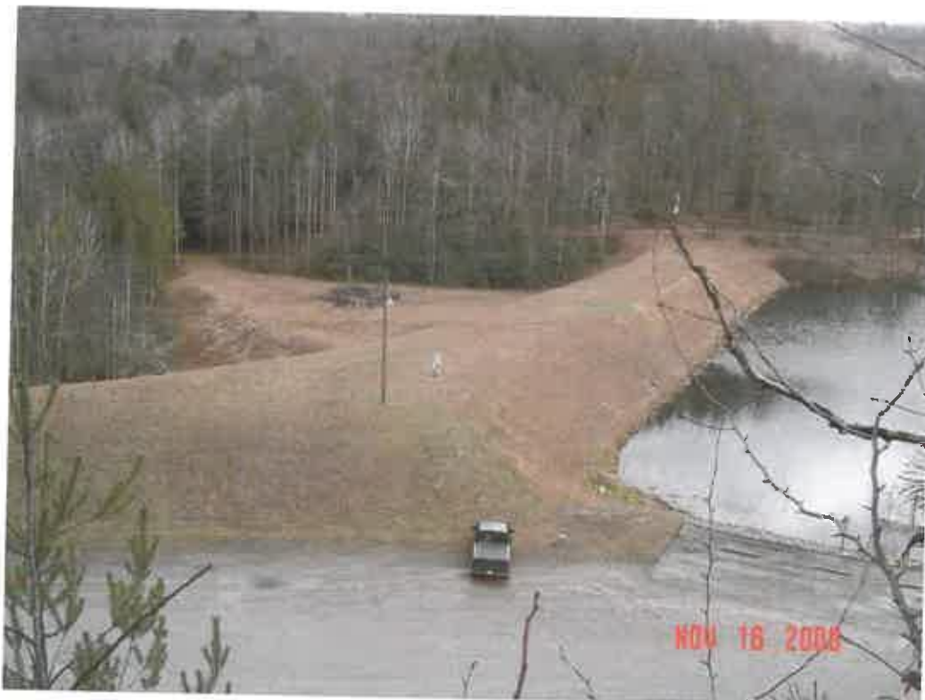
PLUM ORCHARD DAM MODIFICATION, FAYETTE CO., WV
