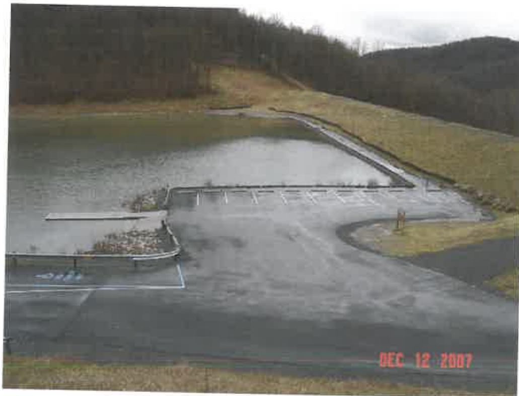
BAILEY DAM MODIFICATION, MONONGALIA CO., WV
