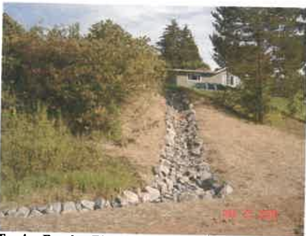
Erosion Repair – Rip Rap Armored Ditch
