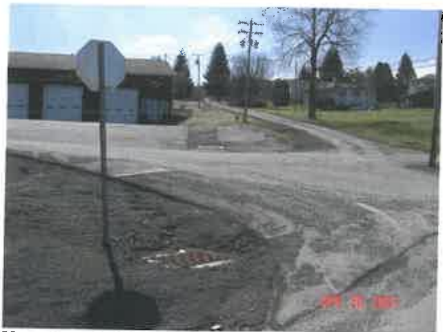
New Storm Drains and Catch Basins
