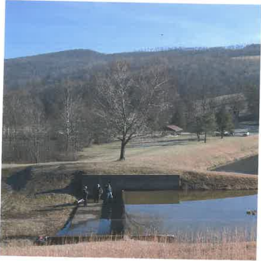
BELINGTON DAM MODIFICATION, BELINGTON, WV
