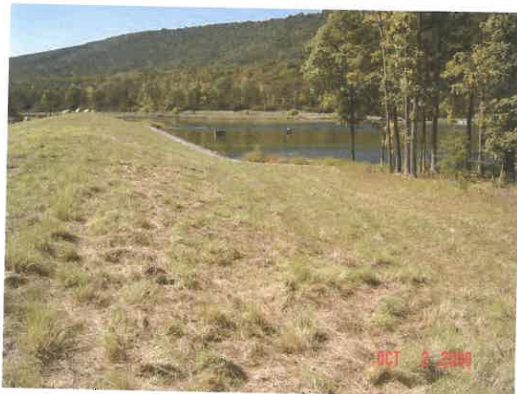
WARDEN LAKE DAM MODIFICATION, HARDY CO., WV
