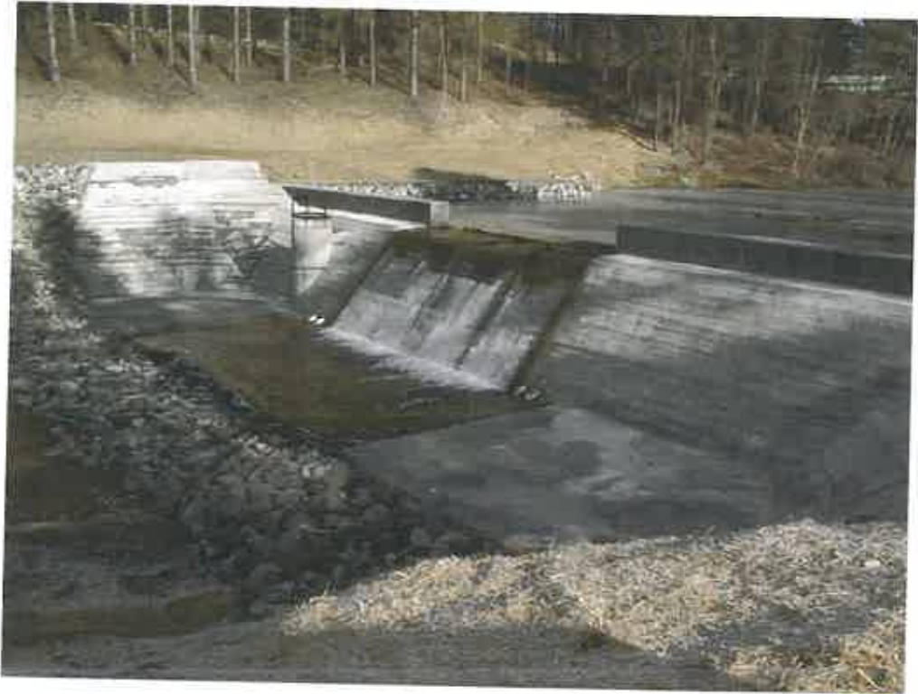
THOMAS DAM MODIFICATION, THOMAS, WV
