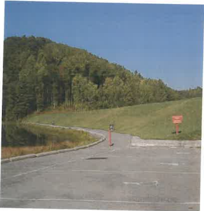
TETER CREEK DAM MODIFICATION, BARBOUR CO., WV
