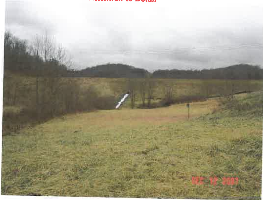
LEMLEY DAM MODIFICATION, MONONGALIA CO., WV
