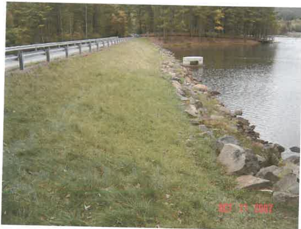
MONCOVE DAM MODIFICATION, MONROE CO., WV
