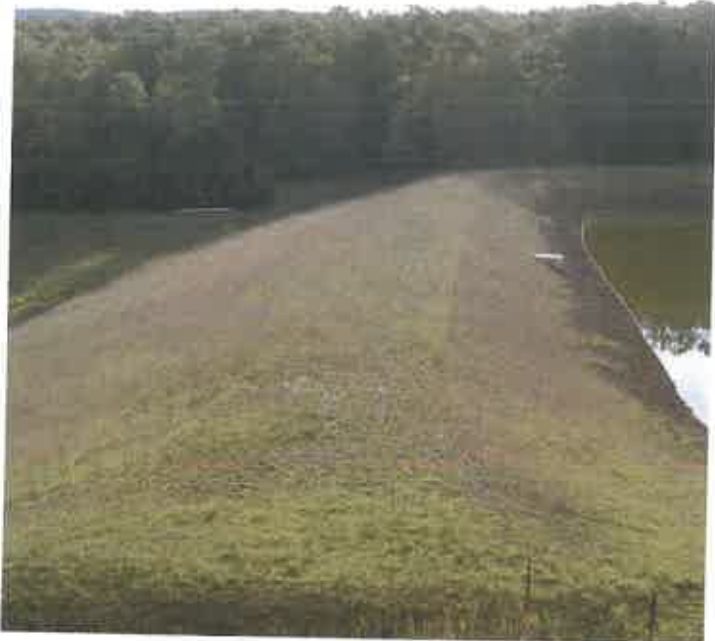
WILSON DAM MODIFICATION, HAMPSHIRE CO., WV
