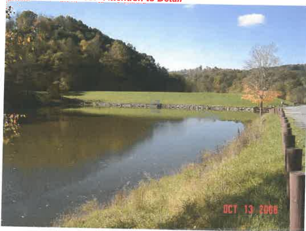
JIMMY LEWIS DAM MODIFICATION, MERCER CO., WV
