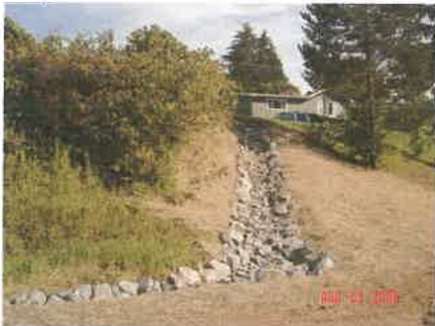
Erosion Repair – Rip Rap Armored Ditch
