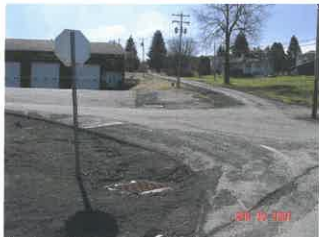
New Storm Drains and Catch Basins
