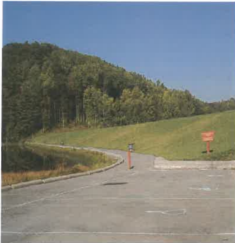
TETER CREEK DAM MODIFICATION, BARBOUR CO., WV
