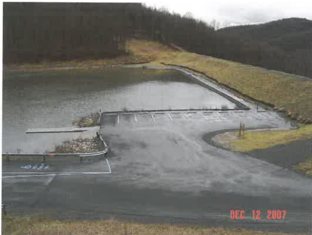
BAILEY DAM MODIFICATION, MONONGALIA CO., WV
