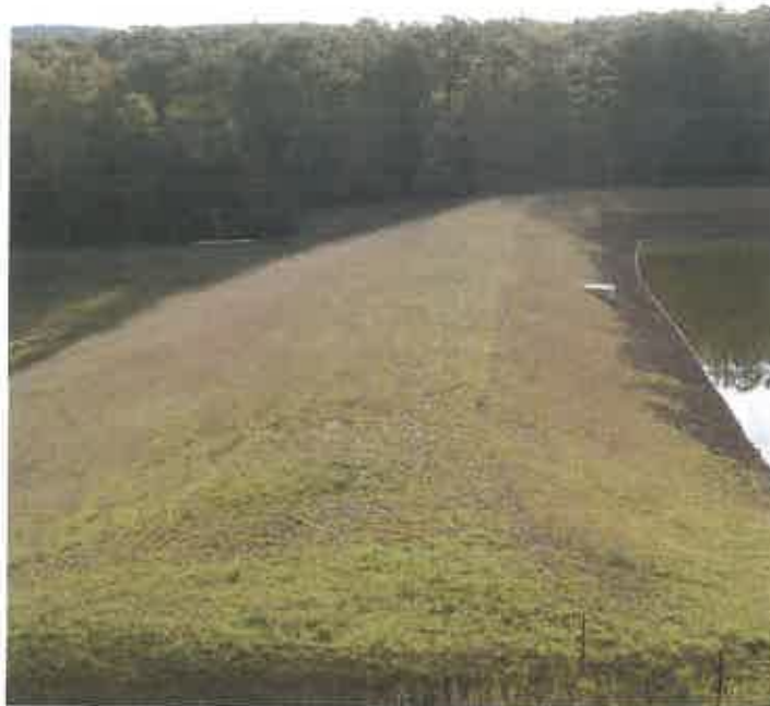
WILSON DAM MODIFICATION, HAMPSHIRE CO., WV
