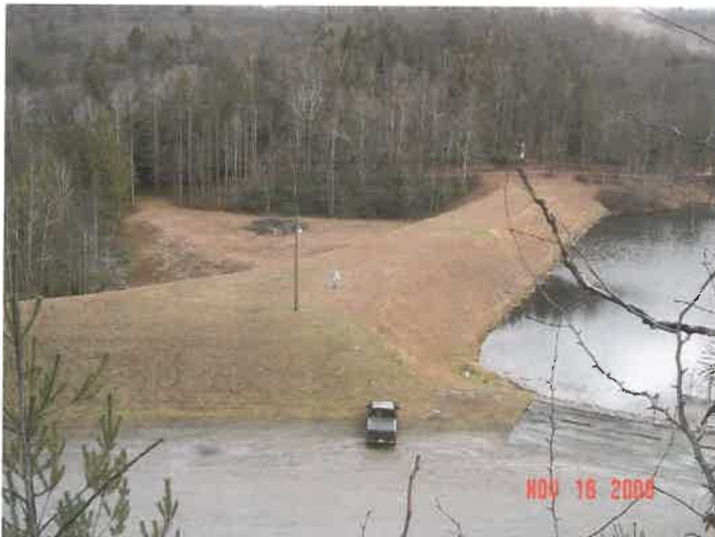
PLUM ORCHARD DAM MODIFICATION, FAYETTE CO., WV
