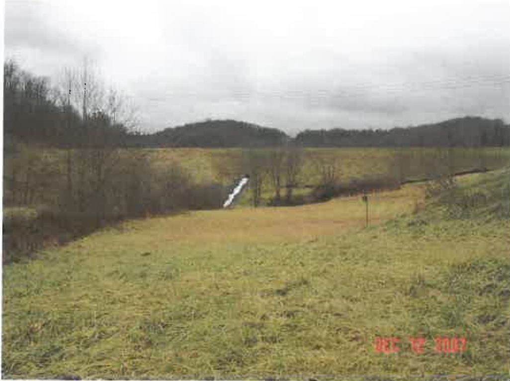
LEMLEY DAM MODIFICATION, MONONGALIA CO., WV
