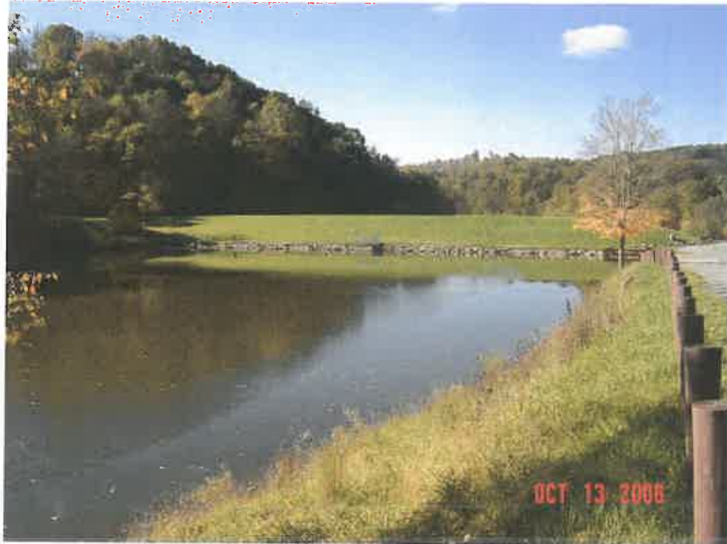
JIMMY LEWIS DAM MODIFICATION, MERCER CO., WV
