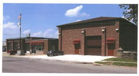
Pickering Associates was hired by the City of Vienna in West Virginia design a new two-story annex to expand a local volunteer fire department's existing fire station facility. The new building contains first-floor pull thru truck bay, conference room, equipment storage and restroom facilities and second-floor offices and storage spaces.
