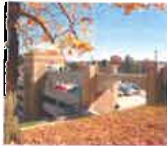
Fairmont State University Parking Garage Fairmont, WV
