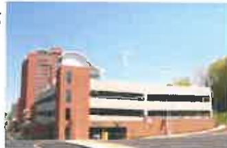
Morgantown Event Center Parking Garage Morgantown, WV
