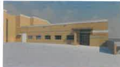
WVUP –New Science Wing- West Virginia University Parkersburg
