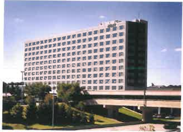
Hyatt Hotel at the Pittsburgh International Airport Dauphin County General Authority Pittsburgh, PA
