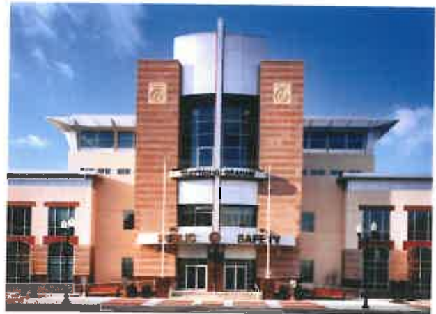
Clayton G. Graham Public Safety Building Atlantic City, NJ
