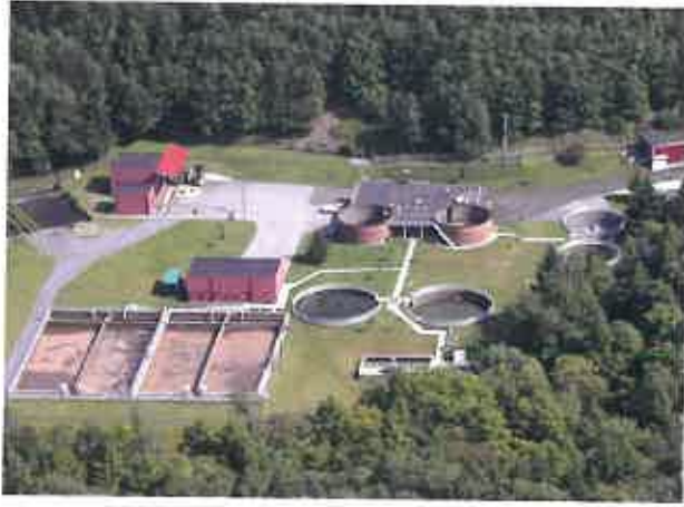
Ebensburg Municipal Authority Ebensburg WWTP Upgrade Cambria County, PA
