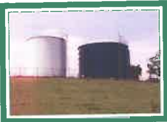
Alderson Water Storage Tanks
