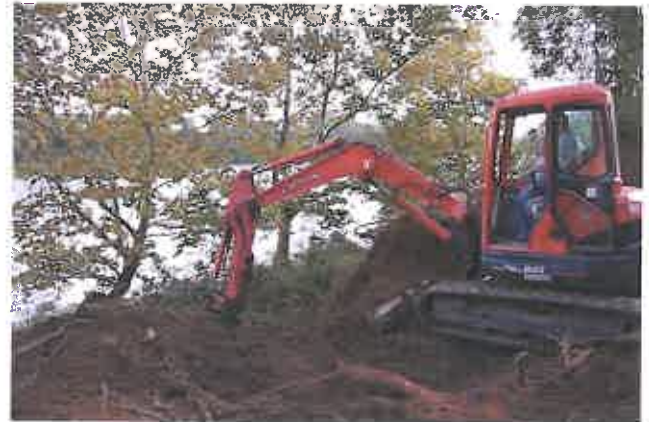
Monitoring of excavator creating trench to accommodate new boat docking facility.
