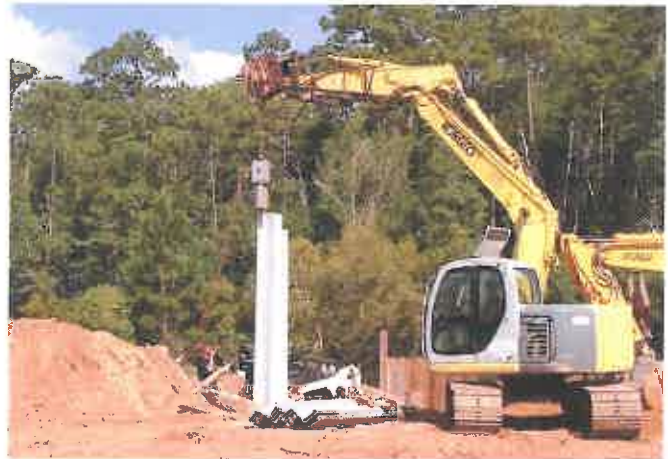
The same proposed Mott MacDonald team also provided construction administration services on the Perdido River boating facility earlier this year.
