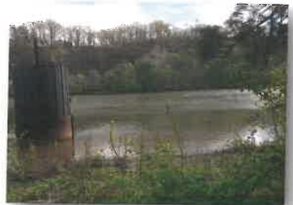
Monongahela River – Project Site Before Construction
