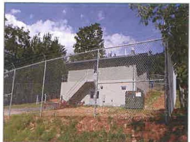
New Water Treatment Plant
