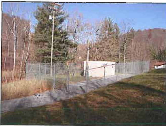
50 GPM Wilsons town Booster Station
