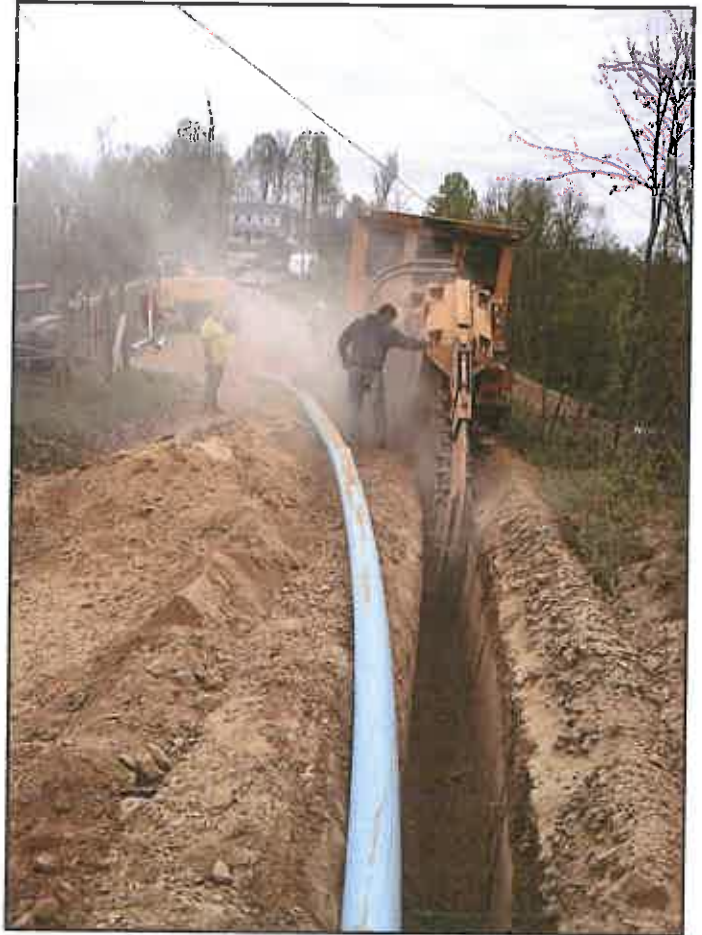
Waterline Installation Along Eight-Mile Ridge Road (Dan's Marine Service)
