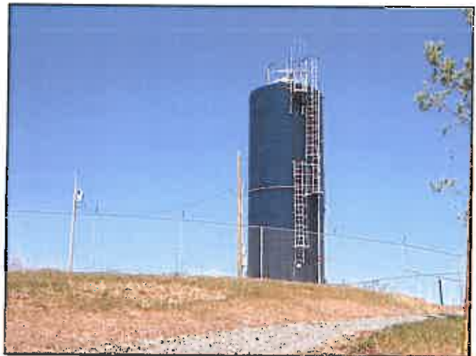
43,000 Gallon Salem Ridge Water Storage Tank
