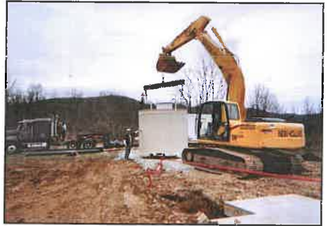
Background – New Master Meter Station Foreground – Foundation for Chemical Feed Station
