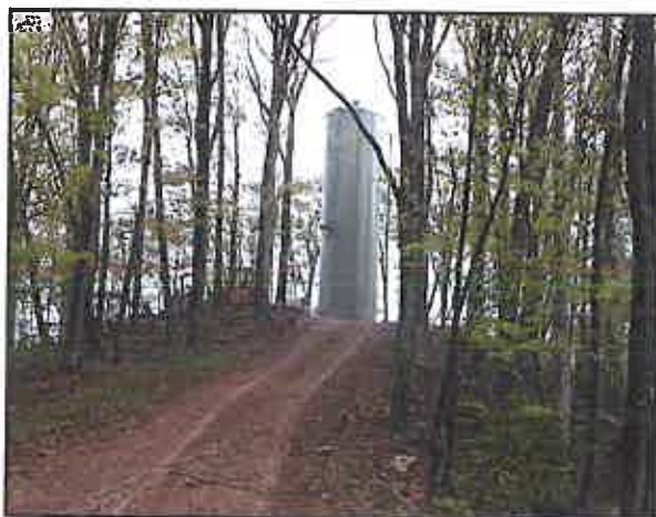
Completed Water Storage Tank
