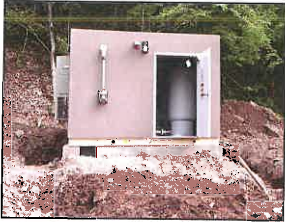
New Hydropneumatic Pumping Station Along Richwood Road
