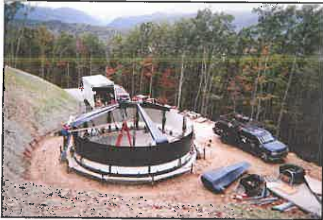
158,000 Gallon Becky's Creek Storage Tank and Site Under Construction
