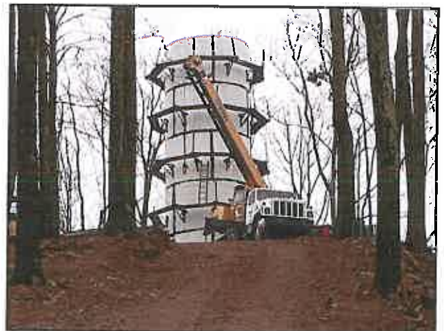
New Water Storage Tank Under Construction
