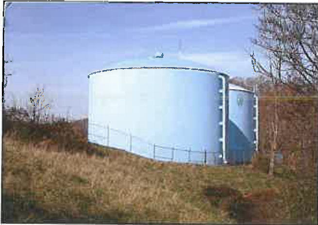
Total Project Cost = $4,400,000 Two 1,000,000 Gallon Storage Tanks Part of FBI Water Project
