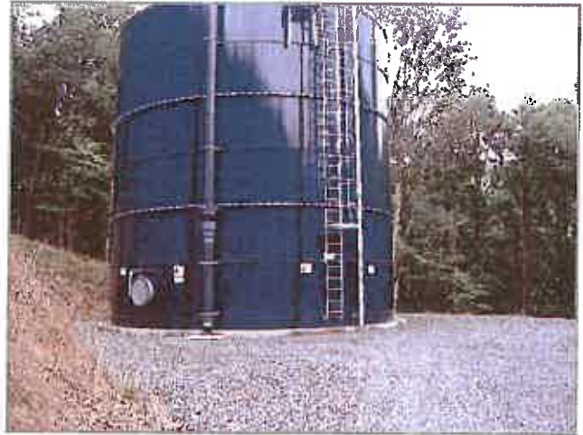
130,000 Gallon Storage Tank Near Valley Head
