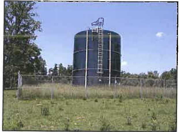
105,000 Gallon Water Storage Tank on Tallmansville Road Near Mt. Carmel Church Road
