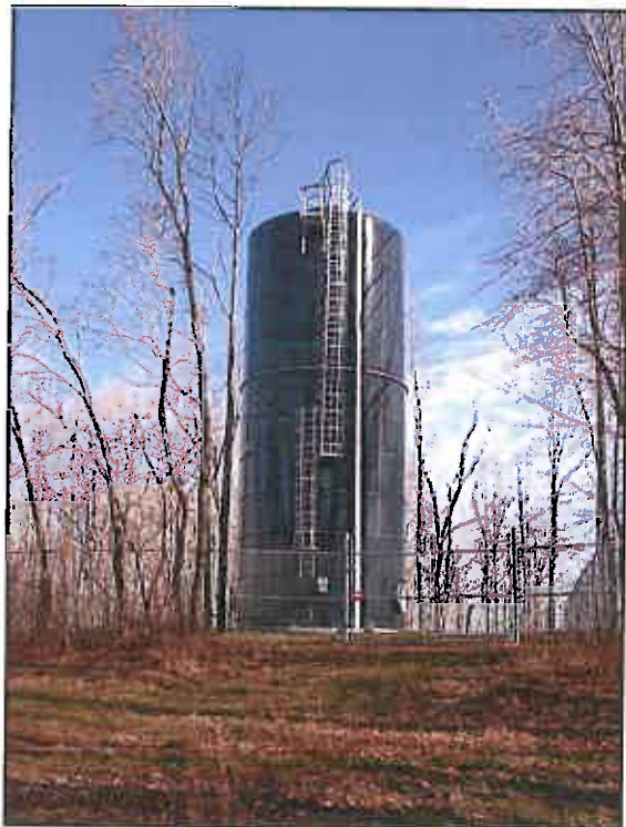
100,000 Gallon Storage Tank on Talbott Road Near U.S. Route 33 (Phase II)
