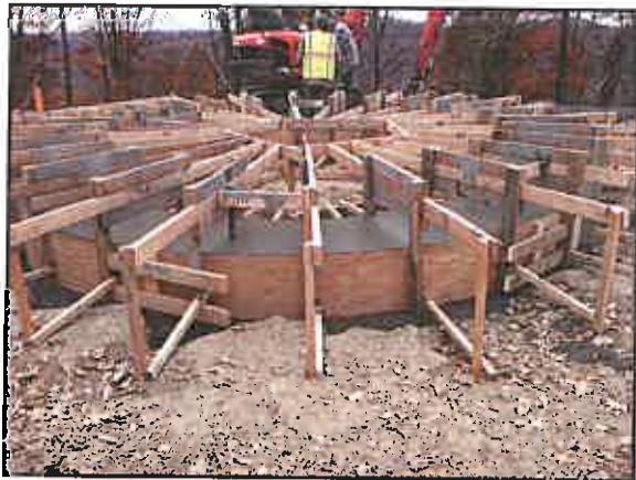
Foundation for New 64,000 Gallon Water Storage Tank (Welding, Inc.)
